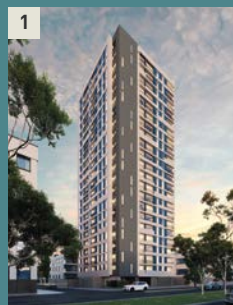
Cor Tower SANTA CATALINA
